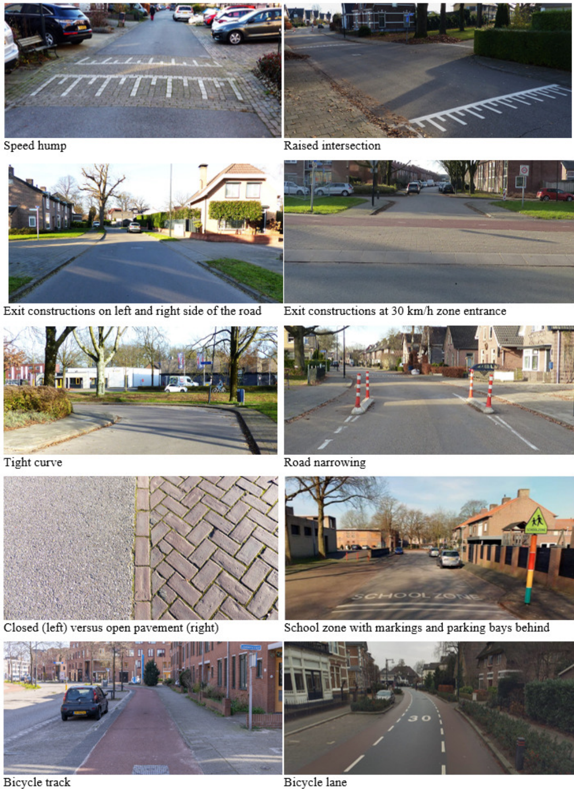
Figure 1. Examples of built environment factors related to driving speed in the Netherlands
