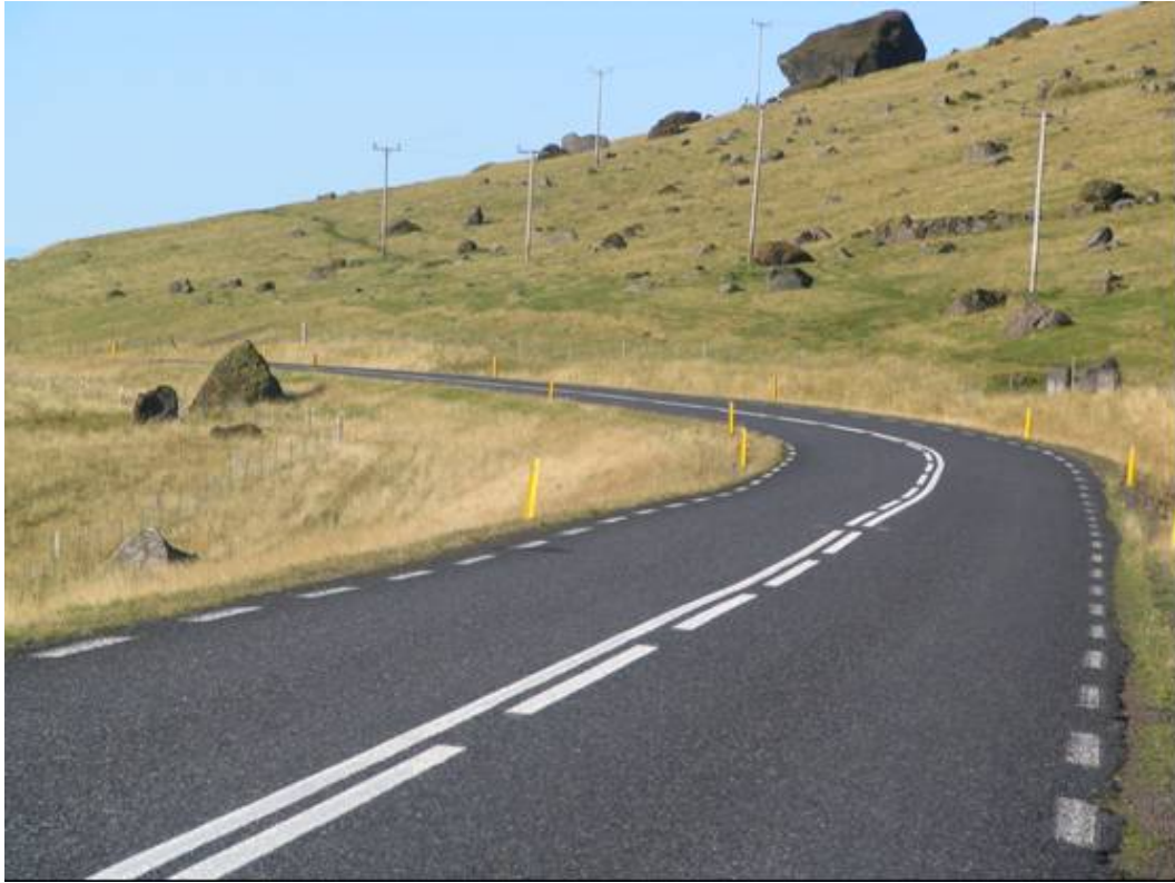
Figure 1 Example of a rock in the roadside (the prominent rock has been removed)
