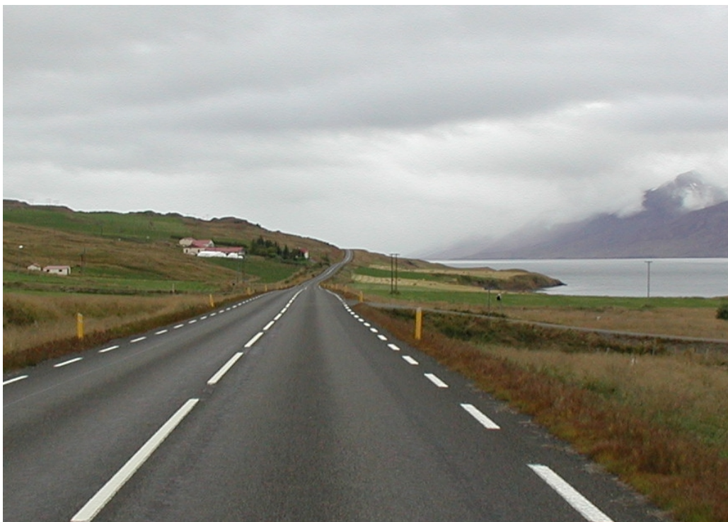
Figure 2 Example of a steep transverse slope on a side road on the right of the main road
