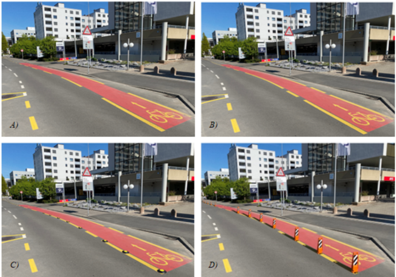
Figure 2 The original colored bicycle lane (A) was supplemented by a continuous line (B), light segregation discs (C) that can easily be crossed, and light segregation with guide beacons (D) that prevent traffic participants from easily riding over them.
