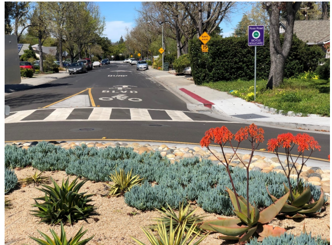
Figure 9 Example from Palo Alto, USA (City of Palo Alto, 2021)
