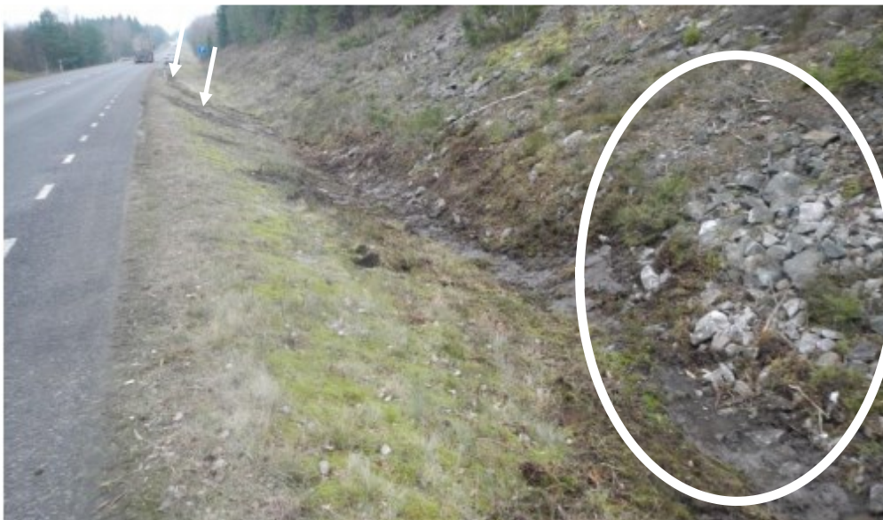
Figure 1. The stones and dirt at a site where a coach with 58 occupants went off the road at 100 km/h because the driver was incapacitated. Photo: SHK (2015)
